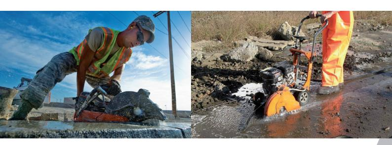
Danterr Diamond Blades are cutting tools with revealed diamond particles arrested in a metal matrix - each with a slight cutting edge. Danterr Diamond Blades are suitable for cutting concrete, pavement, asphalt, roads and even yard pavers and bathroom tiles.
