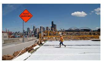
Best applied by spray, however, may also be applied by brush, roller or broom. If the concrete surface is required to be trafficable prior to having an overlay placed, then sand or fine stone can be placed over the Evencure BCP to increase the abrasion resistance of the coating.
