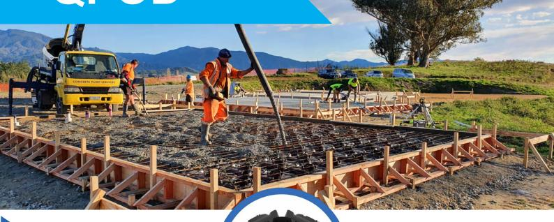
The QPOD™ Flooring System is designed to save the user time while providing an Ecofriendly alternative to polystyrene pods.
