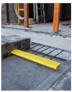
Multiplex Constructions implemented the Nevosafe Rebar Safety Strip at the "The One" tower site on 300 George Street. The same Nevosafe strips introduced at Level 5 are still effectively in use at Level 66 within the Jumpform system. It's well-made, easy to use, and significantly boosts efficiency by replacing 1000+ bar caps with just 30 safety strips. I highly recommend Nevosafe for all steel fixing applications.
